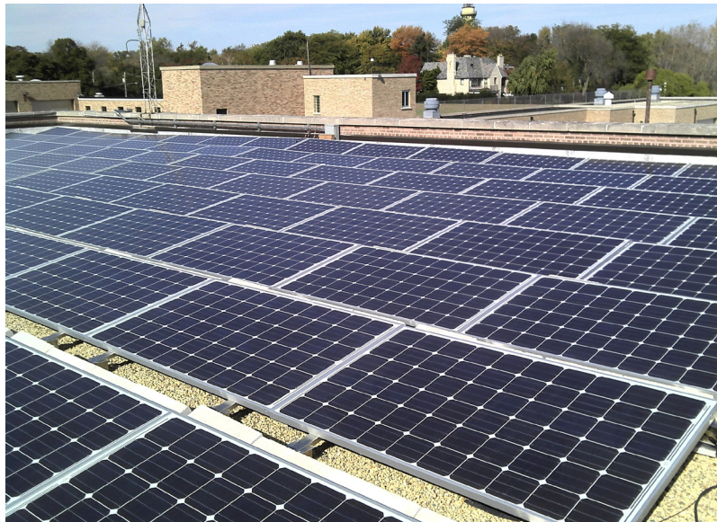
25 kW Array of Solar Panels on Evanston's High Lift Pump Station Roof
