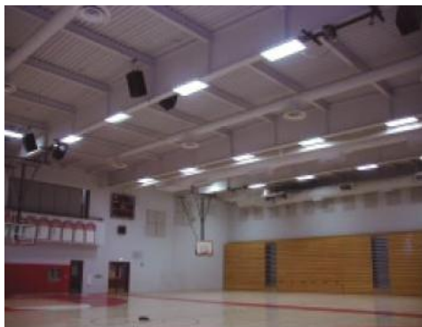
Galt High School upgraded its metal halide fixtures with T5HO linear fixtures, reducing energy consumption by nearly 50%. Photo courtesy of Sacramento Municipal Utility District.
