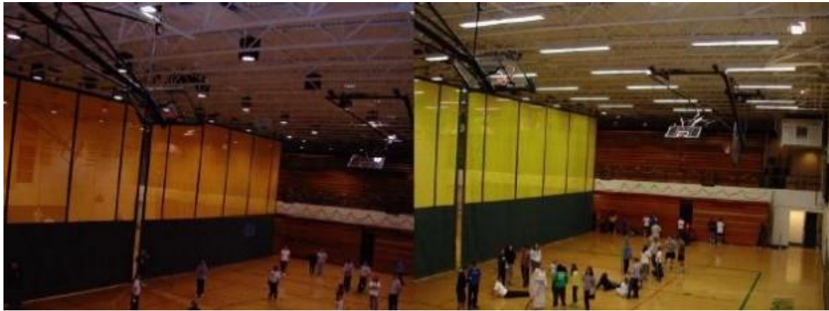
In this school gymnasium, 400W metal halide fixtures (left) were changed over to F32T8 hi-bay fixtures (right) on a one-for-one replacement basis, increasing light levels from 30 to 50 fc and CRI from 65 to 85 while reducing wattage per fixture from 450W to 224W. Photos courtesy of Acuity Brands Lighting.
