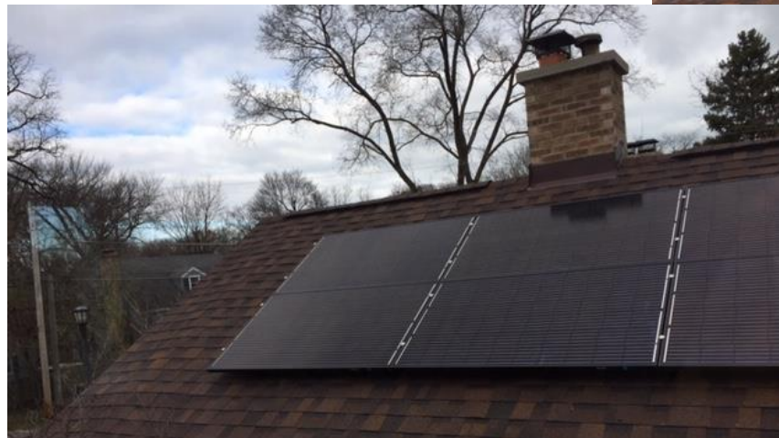
Panels fastened to the rails
