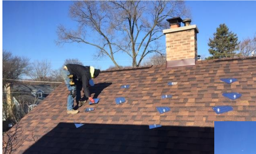
Support “feet” mounted to wood rafters through the roof
