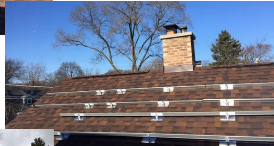
Rails attached to the feet
